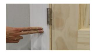
6. **For added support:** remove the center hinge screw from the hinges and replace with a 2" or longer screw (not included). The bracket has a clearance hole for the addition of these screws.
